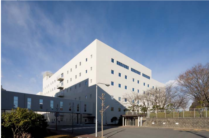
New building of Ashitaka factory
