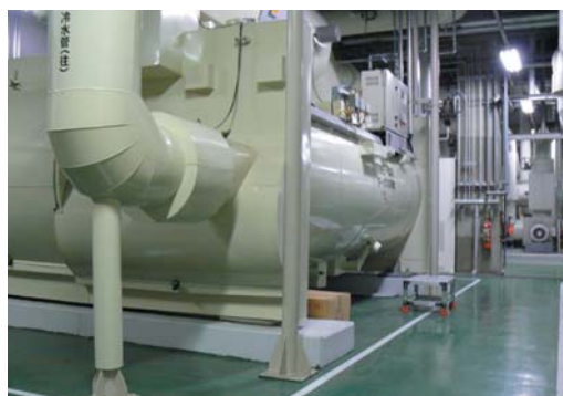
The high-efficiency turbo refrigeration unit (Kofu Factory)
