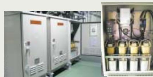
Full view and inside of low-voltage capacitor for improving power factor
