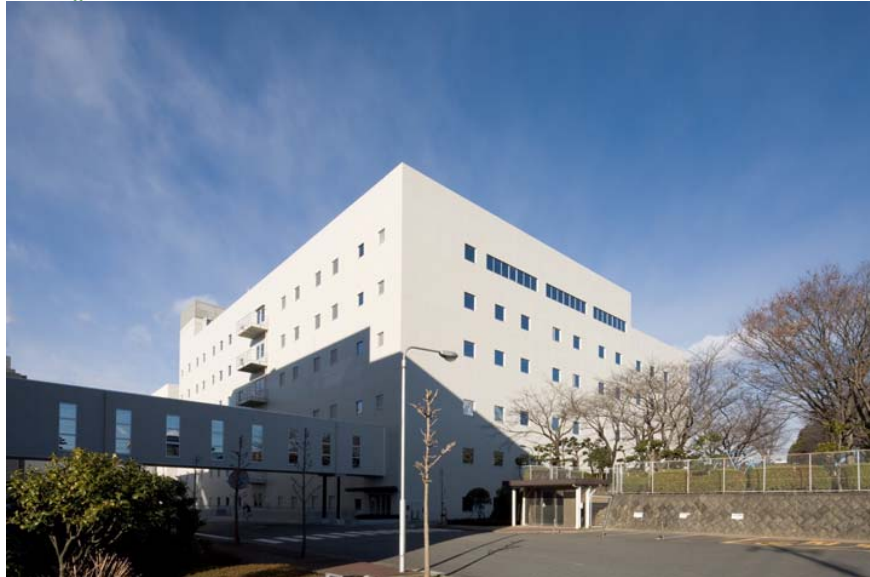
New building of Ashitaka factory
